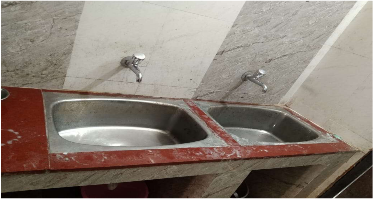
Wash basin installation
